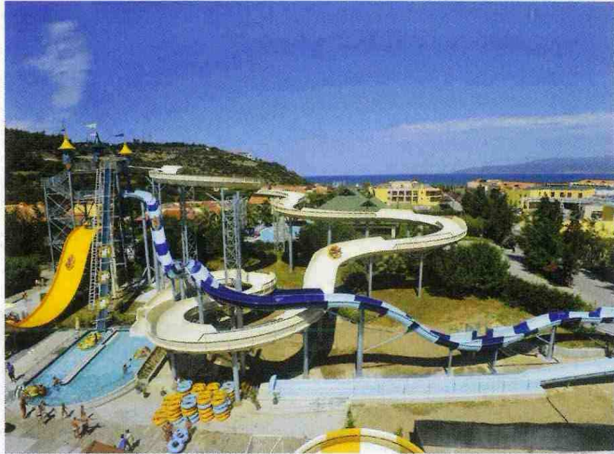
The new 14.7m-high, double-tube slide has twin uphill sections
